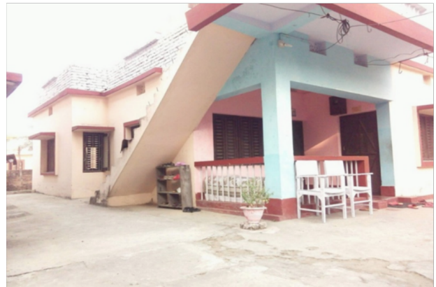
Figure 4: Study building at Biratnagar as viewed from South-East face.
