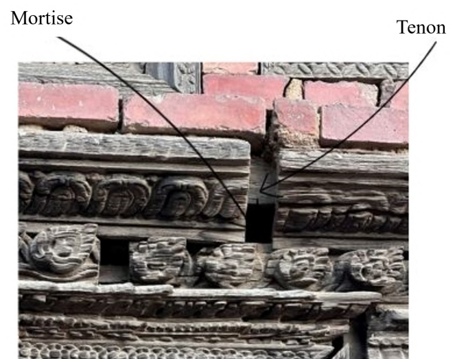
Figure 9: Mortise tenon joint
