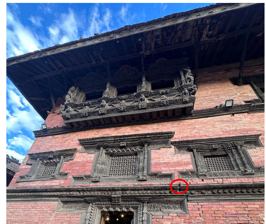
Figure 8: Mortise tenon joint appeared on the historic building of Patan durbar square
