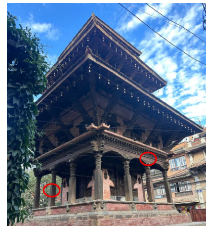
Figure 2: Temple at Swotha square with half lap joint on beam and finger joint on column
