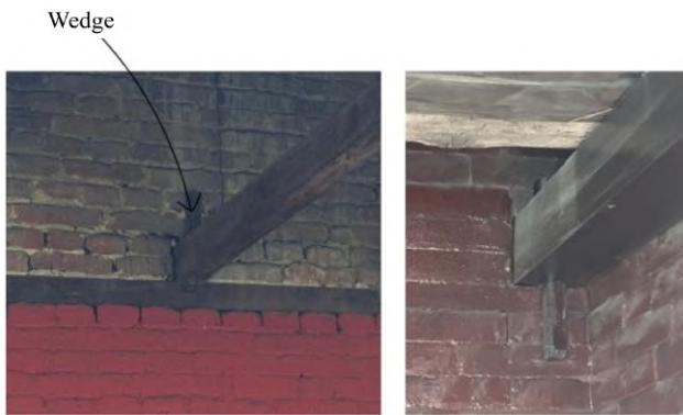
Figure 10: Timber to masonry interface joint
