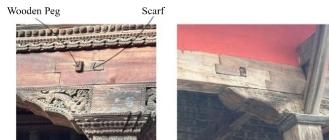
Figure 5: Stop bladed scarf joint with peg
