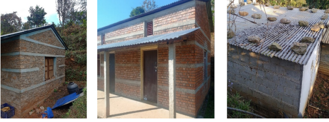
Figure 9: Surveyed houses of stone in cement, brick in cement and hollow concrete material.
