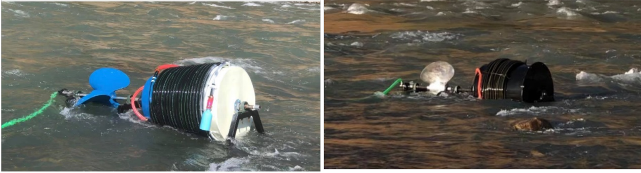
Figure 6: Installation of two pump in Sunkoshi river, Nepalthok, Sindhuli.
