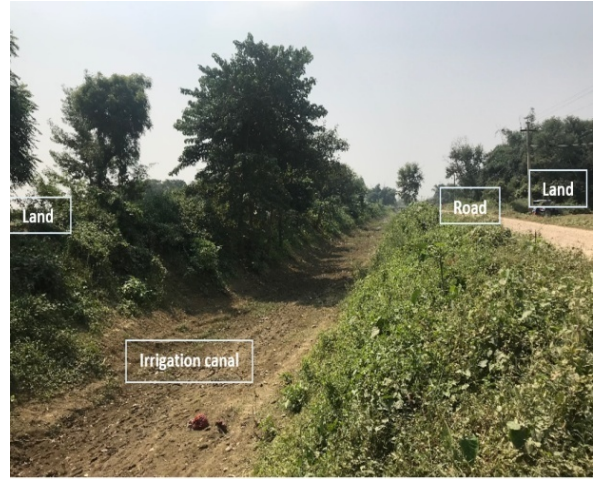
Figure 1: Irrigation canal in Bara.
