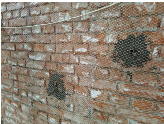
Figure 16: Retrofit of wall using wire mesh and cement grouting
