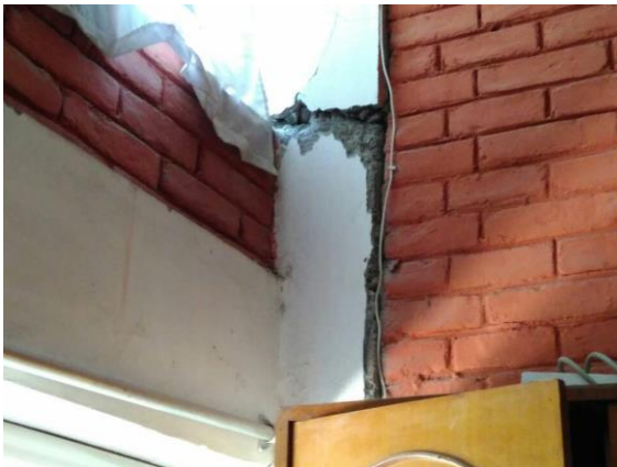
Figure 9: Short Column/Captive column Effect
