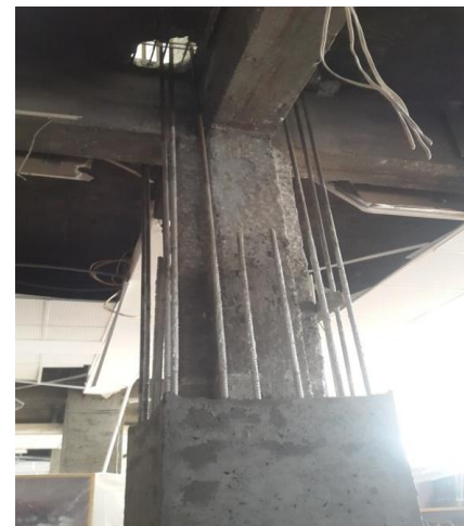
Figure 17: Retrofit of column by jacketing method.
