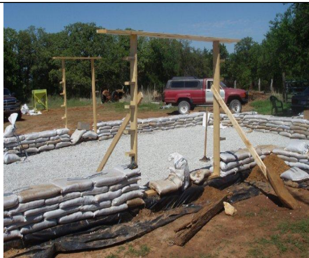
Figure-3- Earthbag Construction
