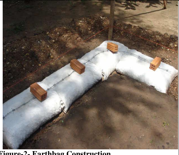
Figure-2- Earthbag Construction
