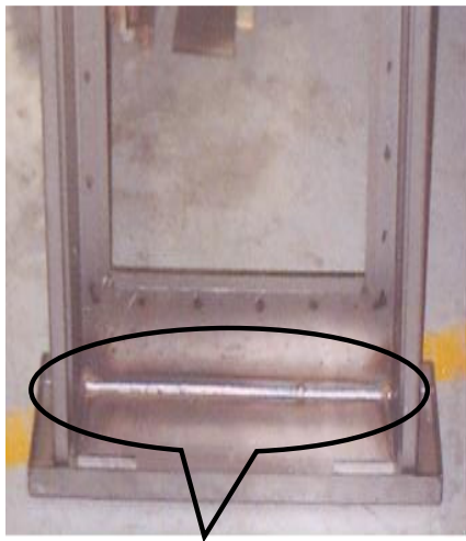
450 mm horizontal fillet welding
