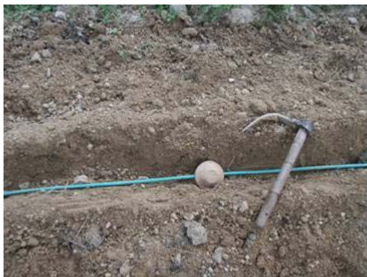
Plate 3. Sub-surface installation of drip-irrigation pipe.
